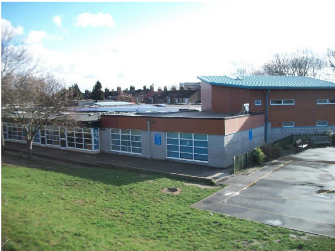
Existing School Building
